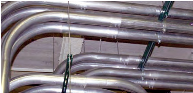
Faster EMT Installations
